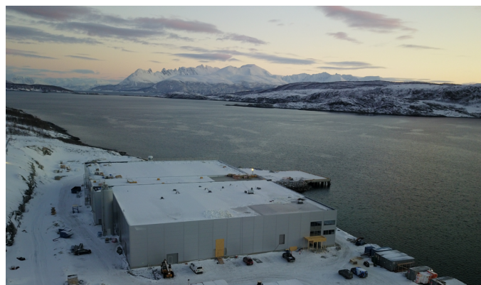
The new freshwater facility at Sandøra
