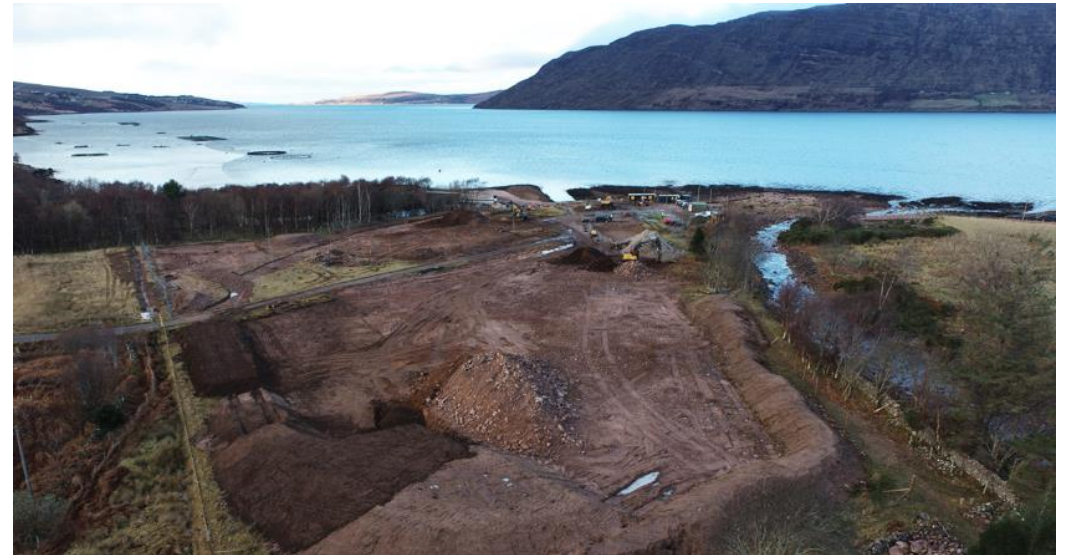
Construction has commenced (above). Groundworks (below). Ardesie, Scotland.
