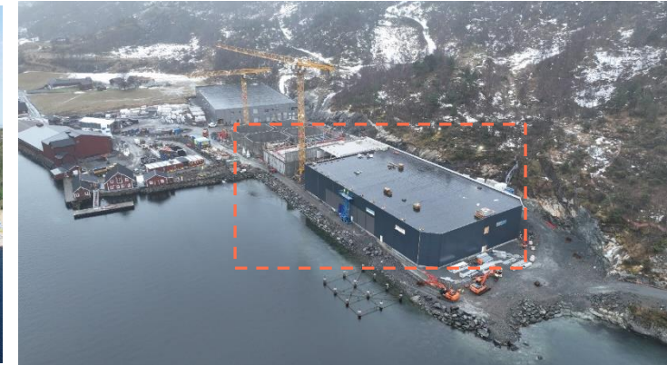
Norway - Haukå commissioning Q4-24
