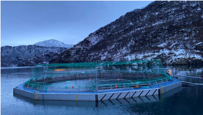
Norway - Closed Containment System
