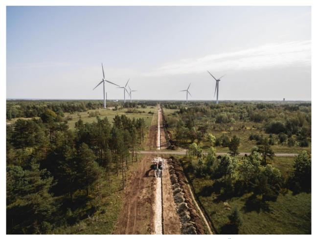
Earthworks on the Kiili-Paldiski section of a DN700 MOP54 gas pipeline. Kaurits OÜ
