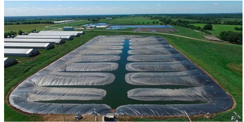
Smithfield manure lagoon for renewable natural gas production
