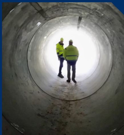
Valby cloudburst tunnel Copenhagen
