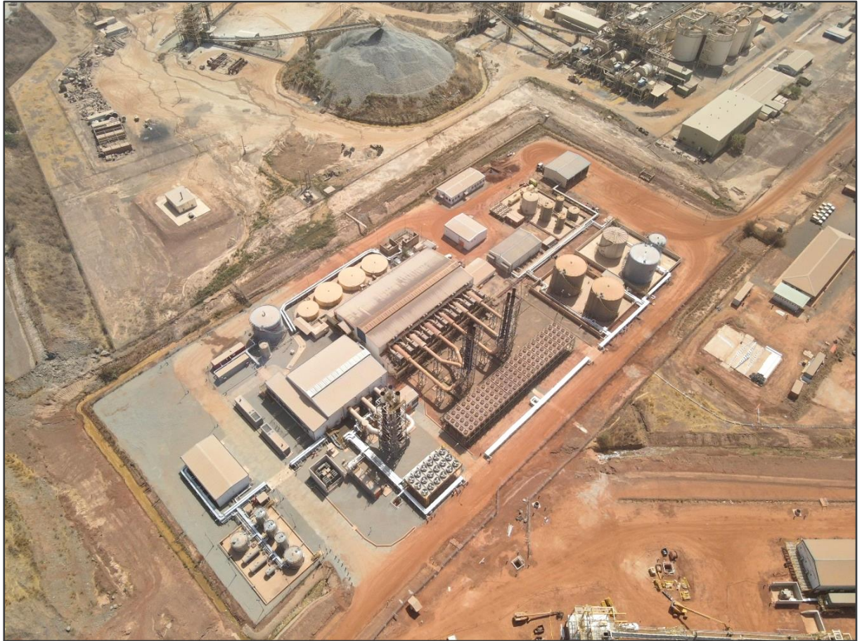
Figure 11: 18MW HFO power plant expansion was completed and successfully energised during Q4-2023, increasing the capacity of the existing power plant by 50%
