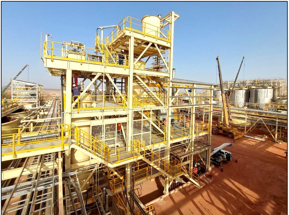
Figure 8: Elution and electrowinning circuit construction is largely complete with wet commissioning planned for early March
