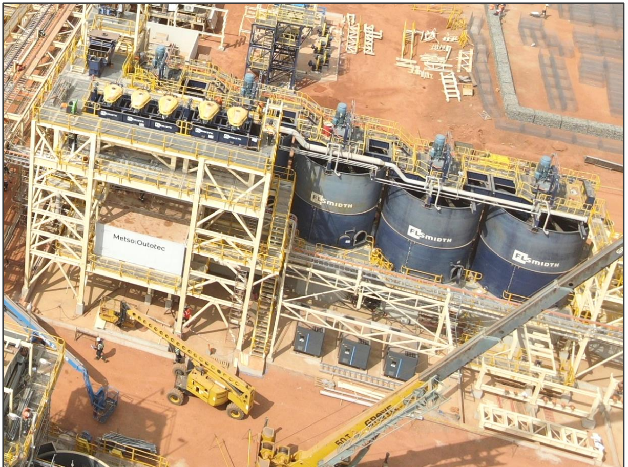
Figure 4: Flotation circuit construction is largely complete and sulphide concentrate is expected to be delivered to the BIOX ® circuit in early March
