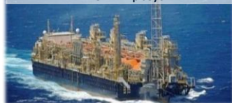
FLNG Gimi (under construction)
