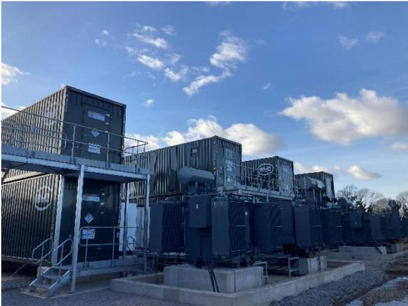
Located at Avonmouth, near Bristol, Hallen BESS is a lithium-ion battery storage facility comprising 16 modules, each with a capacity of 2 megawatthours per unit. Initially scheduled for the first quarter of 2022, the plant stored and then released its first kilowatthours on December 23, 2021.
