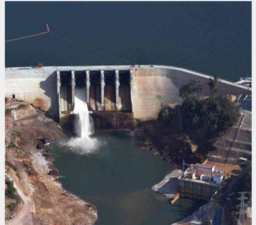
THPC 525 MW hydro power plant
