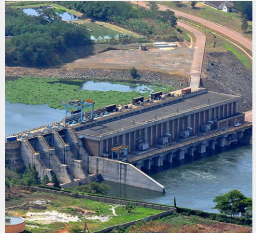
Bujagali 255 MW hydro power plant
