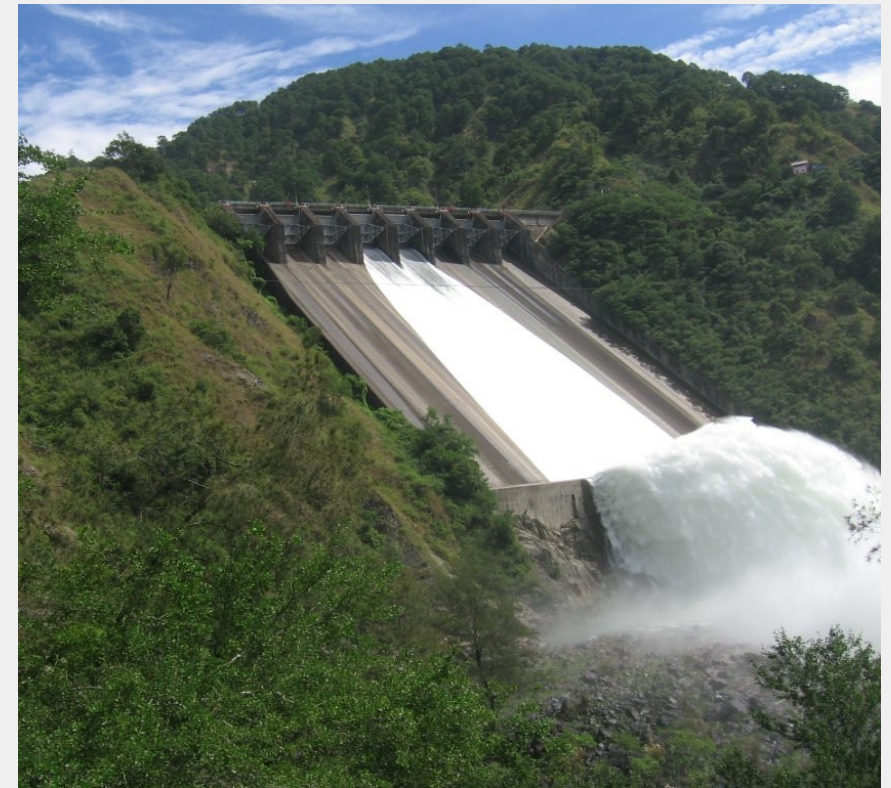
Binga 140 MW hydro power plant
