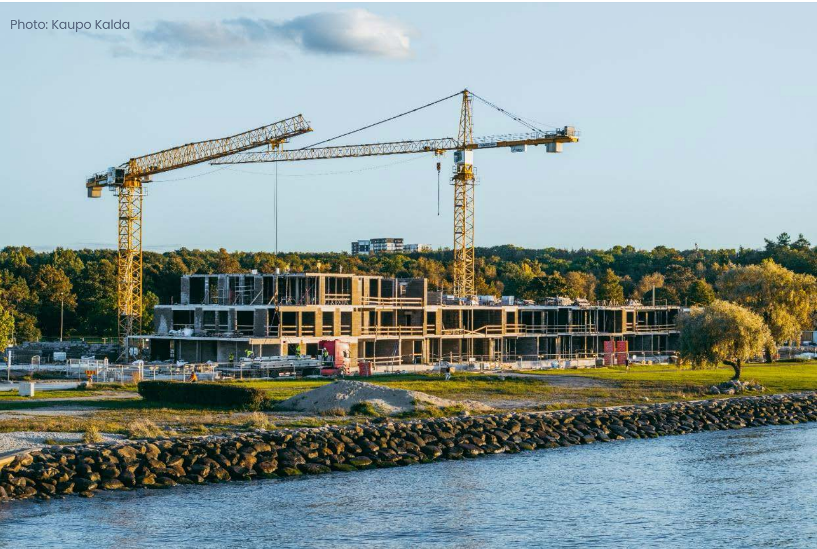
Construction of phase I of the Regati development
