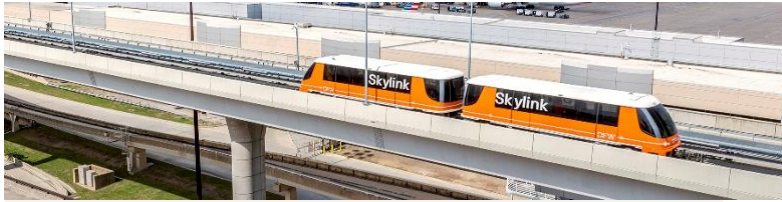
DALLAS (10 YEARS OPERATION & MAINTENANCE – US)
