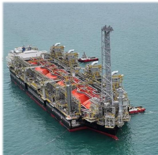
FLNG Gimi (ready for operations) - MKI (2.7mtpa)
