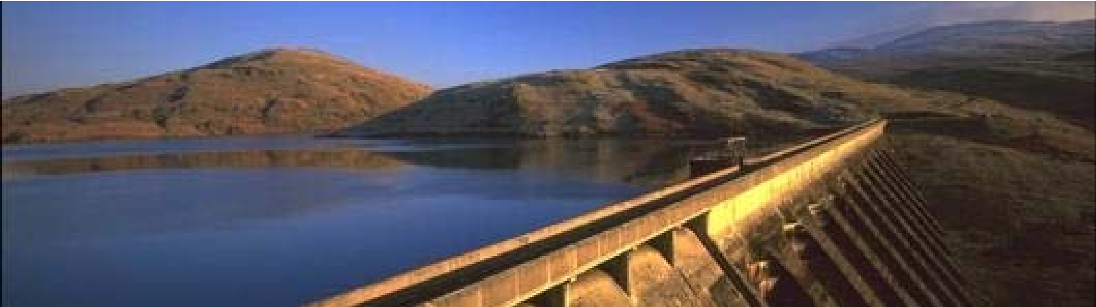
Rheidol hydropower plant, Wales
