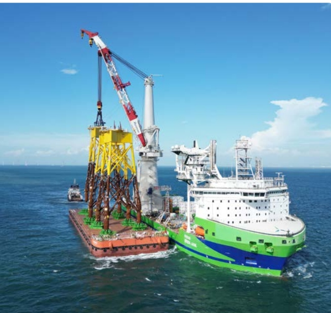
DEME • Offshore Energy, Zhong Neng
