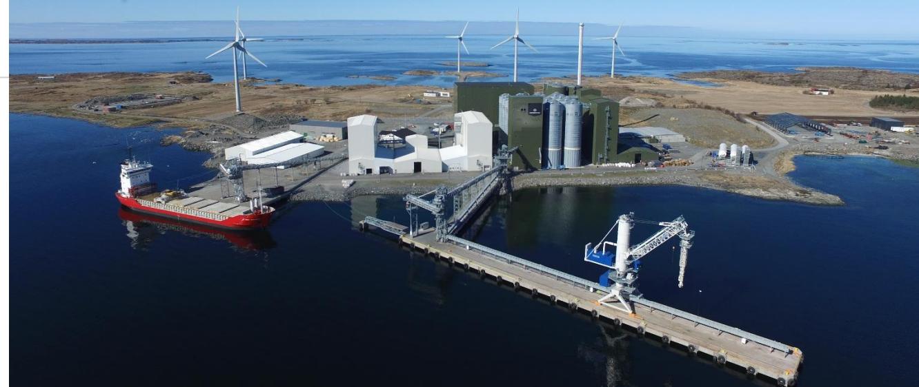
Scotland: New plant
