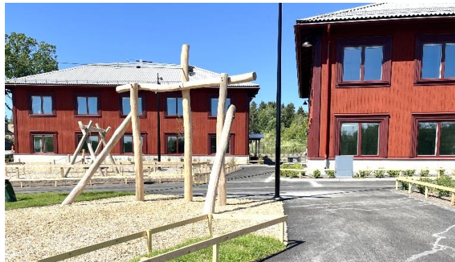
Nynäshamn Källberga in Nynäshamn (SE) School completed in July 2024
