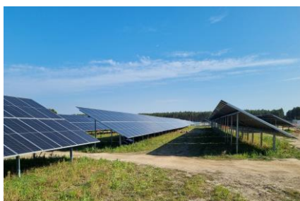
PV Energy Projects, Zaganiec construction site.
