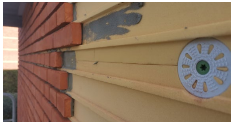
Tinby Skumplast supplies insulation sheets to Briiso for their façade insulation system.
