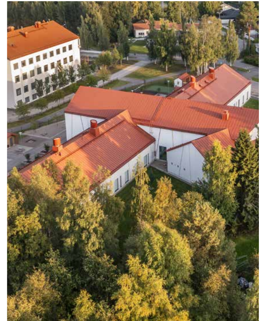
OULU VALJASTIE - CHILDCARE CENTRE IN OULU (FI)
