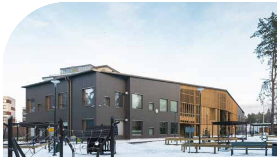
HELSINKI KUTOMOKUJA - CHILDCARE CENTRE IN HELSINKI (FI)
