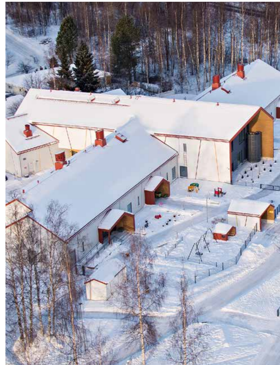
OULU VALJASTIE - CHILDCARE CENTRE IN OULU (FI)
