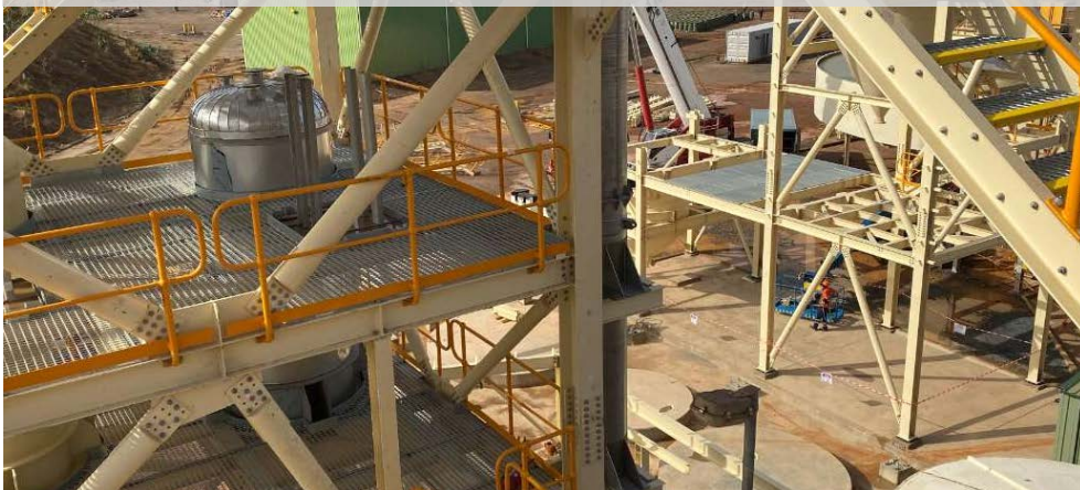
Package 3: Additional acid wash and elution column: staircase and grid mesh installation
