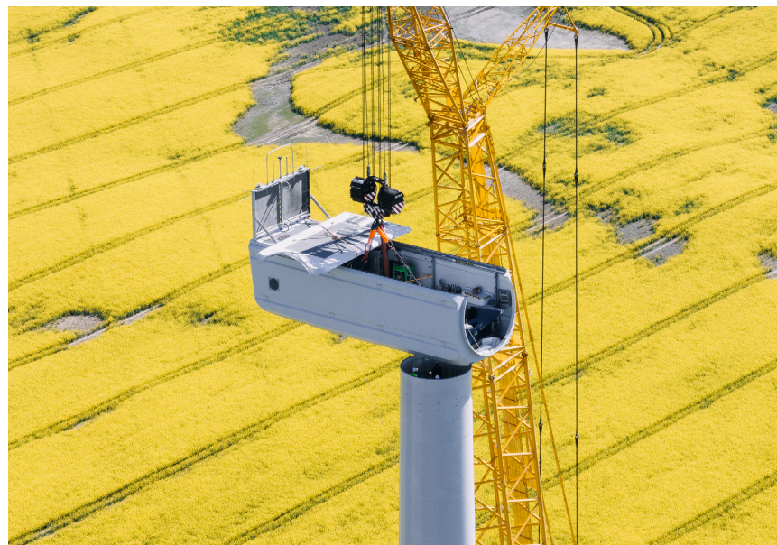
Construction of the Kelmė WF in Lithuania
