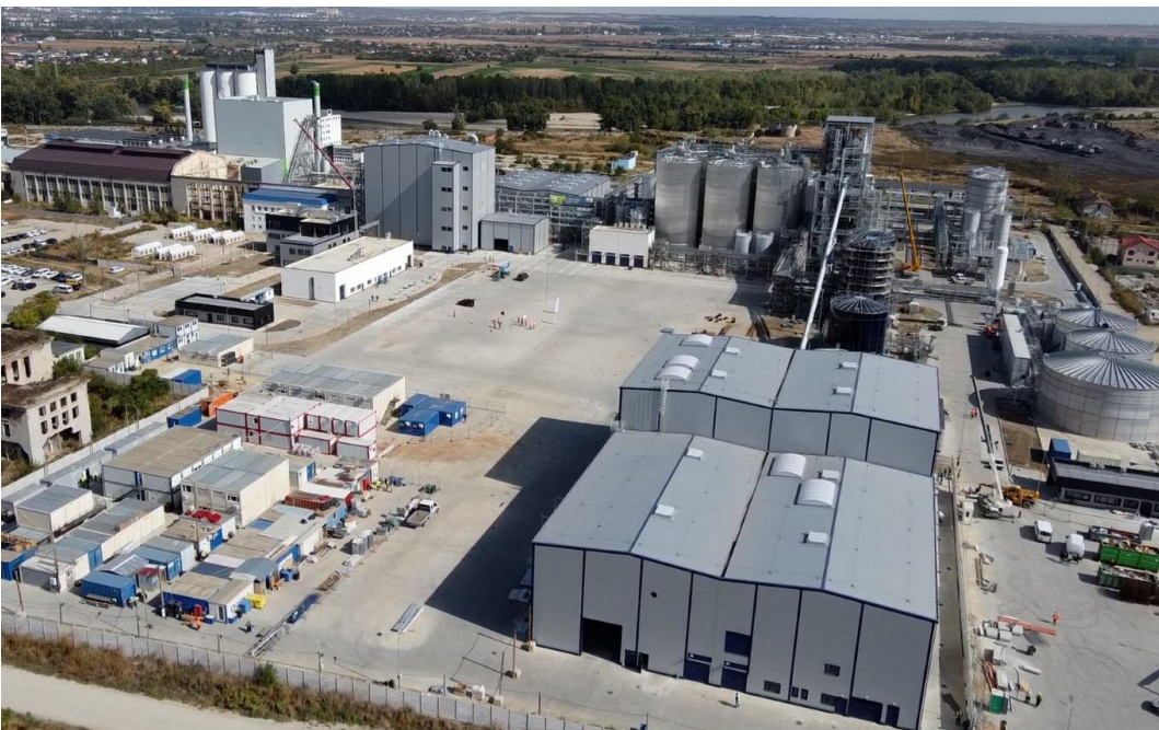
Clariant’s flagship commercial sunliquid® cellulosic ethanol plant in Romania. (Picture: Clariant)
