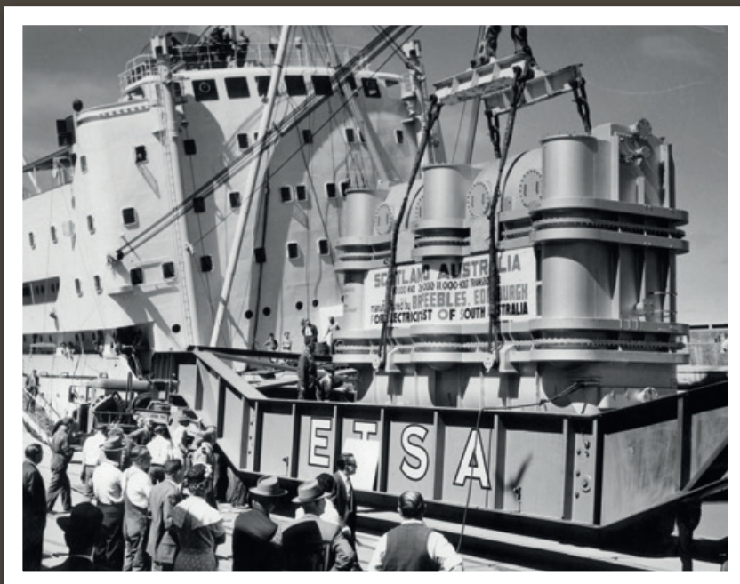
Transformer underway from scotland to australia
