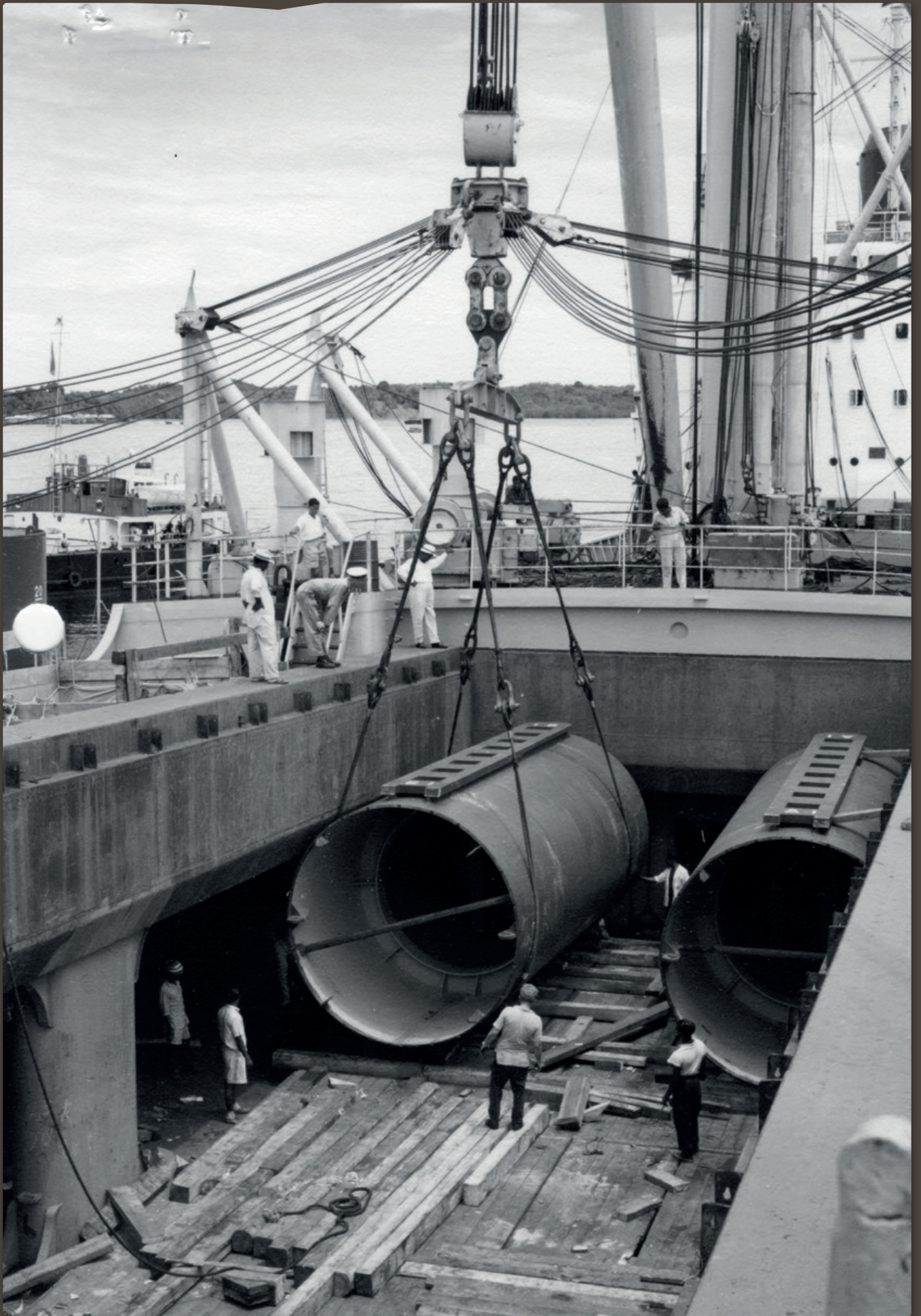
Transformer underway from scotland to australia. 1949
