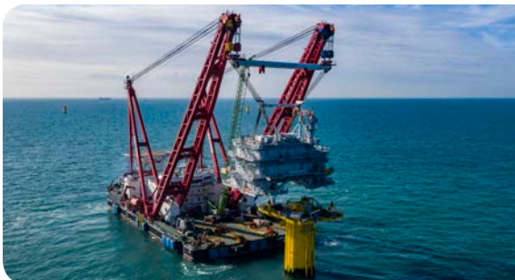
DEME - SeaMade - Installation of offshore substations
