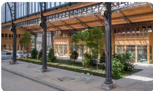
Extensa - Tour & Taxis - Gare Maritime - Brussels
