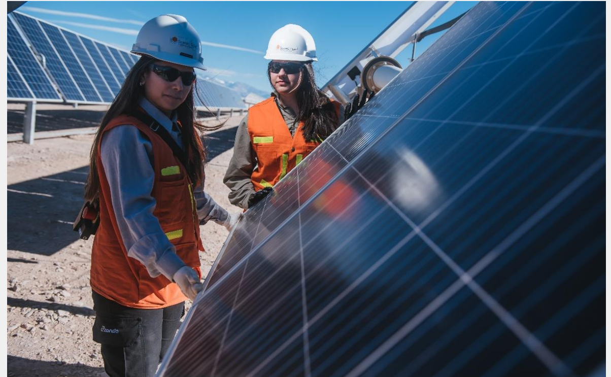
Installation of solar panels at the Guañizuil IIA project, Argentina.
