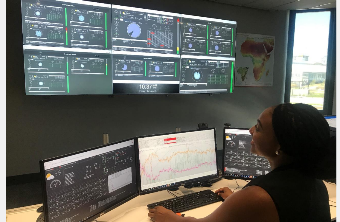
Scatec Solar's 24/7 global Control & Monitoring centre in Cape Town.
