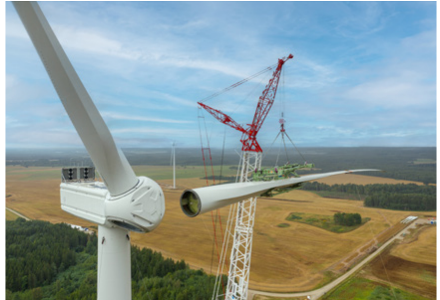
Construction of the Mažeikiai wind farm in Lithuania
