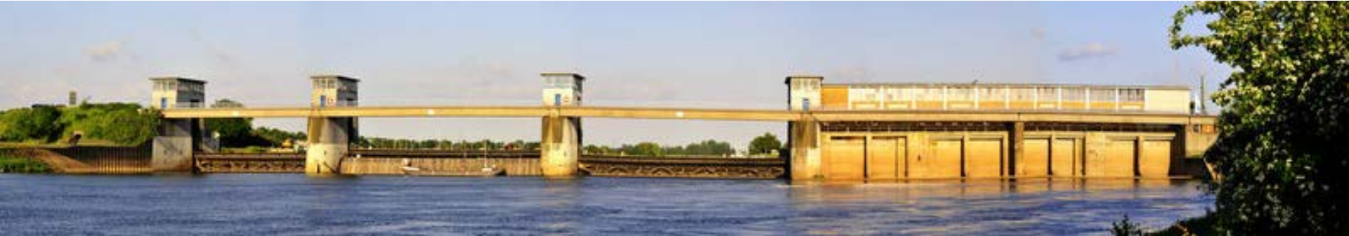
Dörverden hydropower plant, Germany
