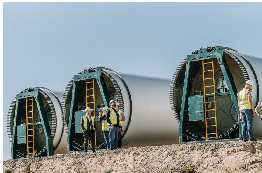
Construction of the Kelmė WF in Lithuania
