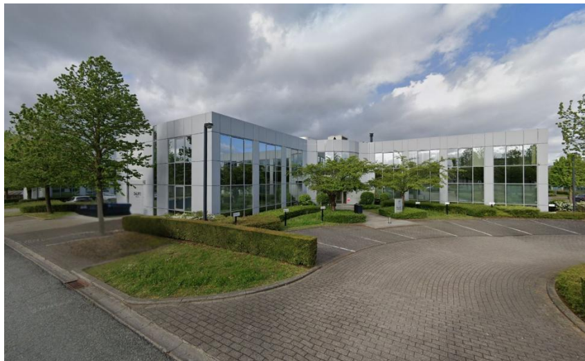
THEON Production Facility within IKAROS Park, Zaventem, Belgium
