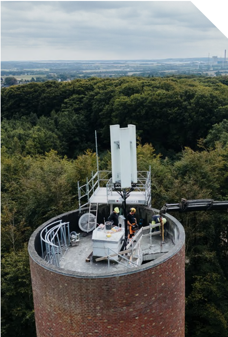
MT Højgaard Denmark employs drilling and cutting specialists both on Zealand and in Jutland. Here they help cut holes through the water reservoir in a water tower in Vodskov.
