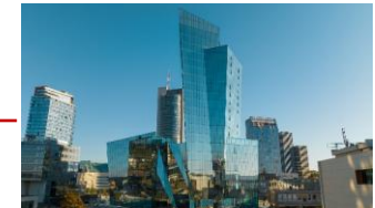
Artery Business Centre Completed in 2023
