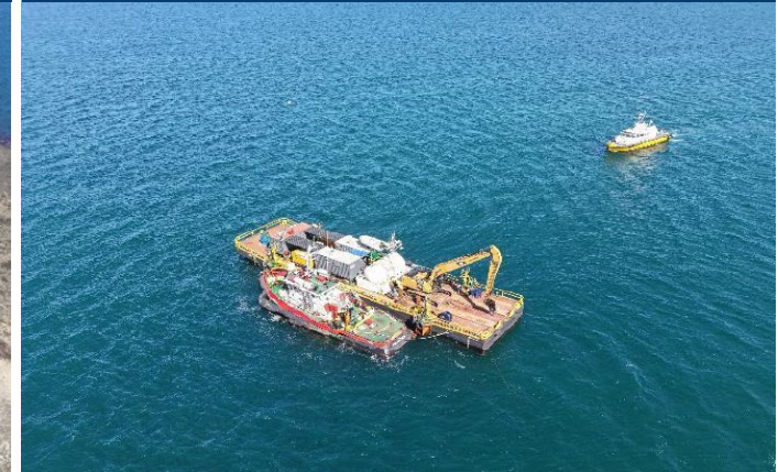
Trenching activities for 2 x 5km offshore pipelines to FLNG mooring sites
