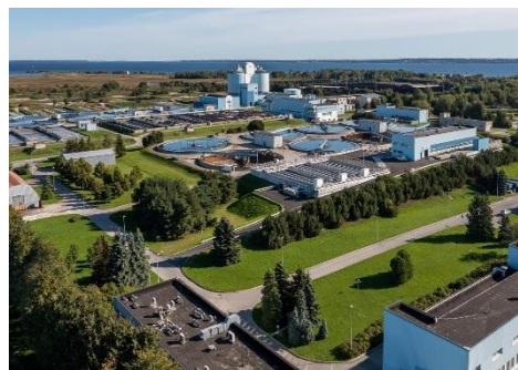
Paljassaare Wastewater Treatment Plant
