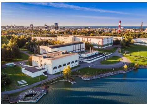
Ülemiste Water Treatment Plant
