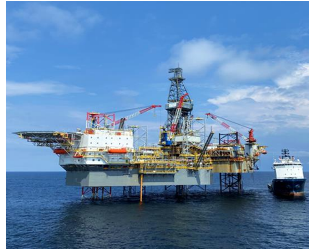
BW MaBoMo drilling operations on the Hibiscus / Ruche development
