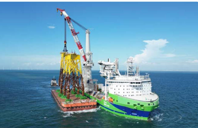
DEME • Offshore Energy, Zhong Neng
