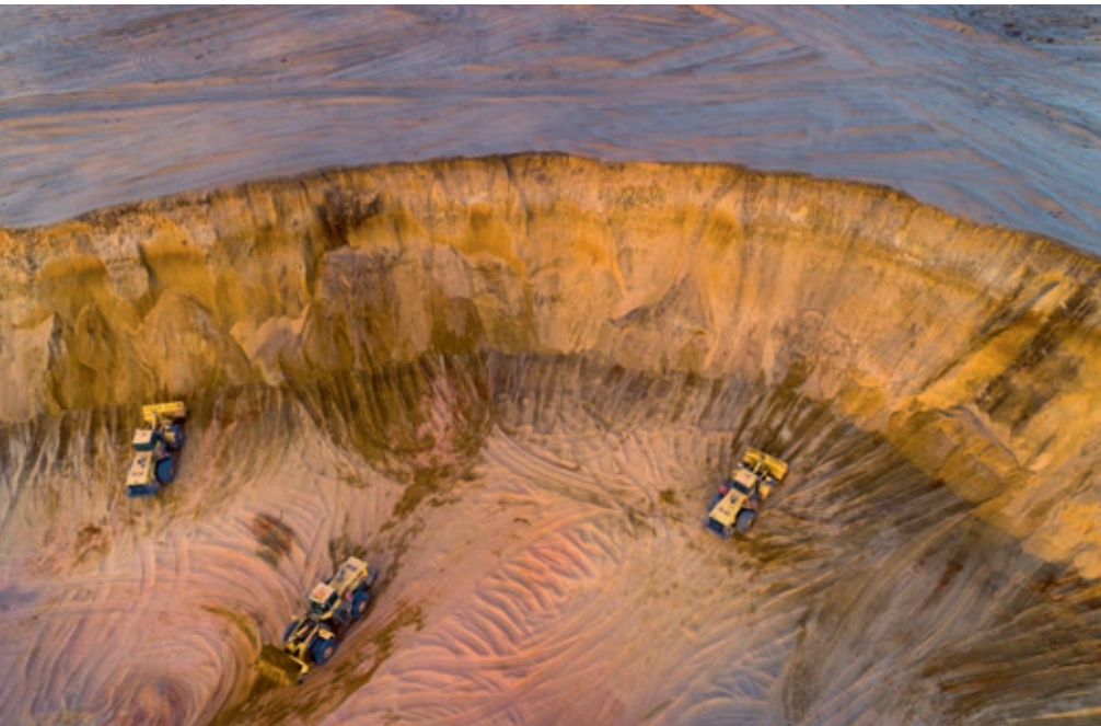
Image: Aerial view of dry mining being conducted by front-end loaders and their operators at the Mine.
