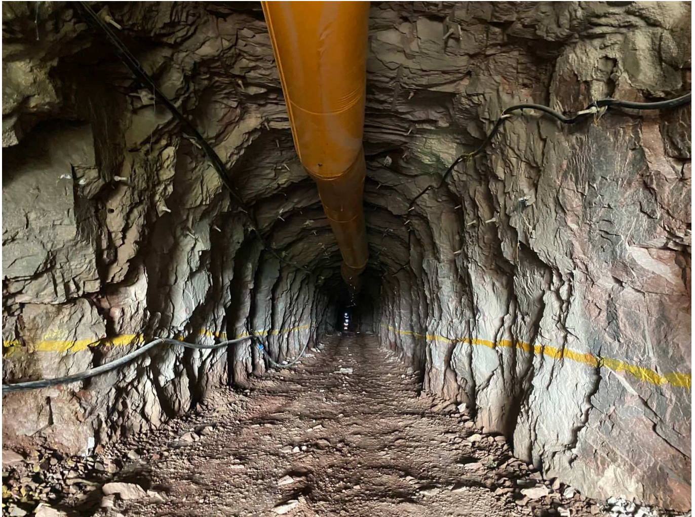
Figure 7 – The Serra Ramp Established
