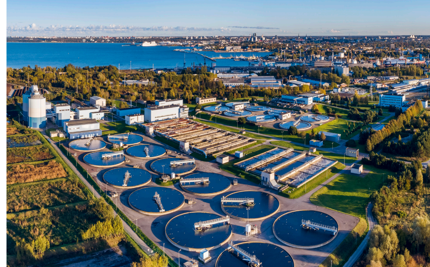
Paljassaare Wastewater Treatment Plant
