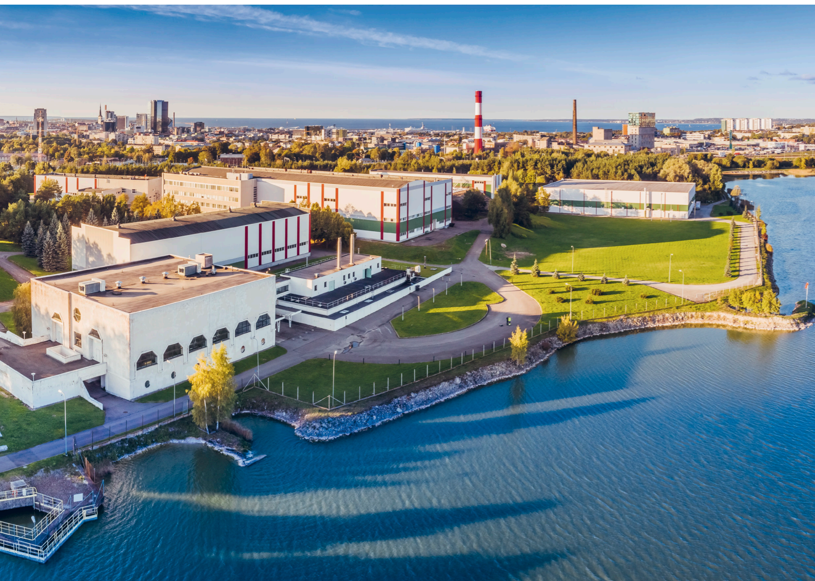
Ülemiste Water Treatment Plant
