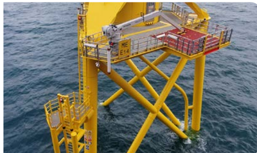
DEME - Moray East - First jacket foundation
