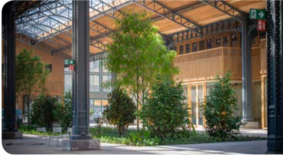
Extensa - Gare Maritime - Tour &amp; Taxis
