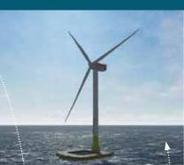
Capacity: 30MW / 3 units Water depth: 55 metres
