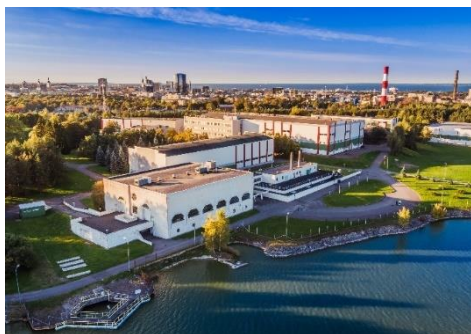
Ülemiste Water Treatment Plant
