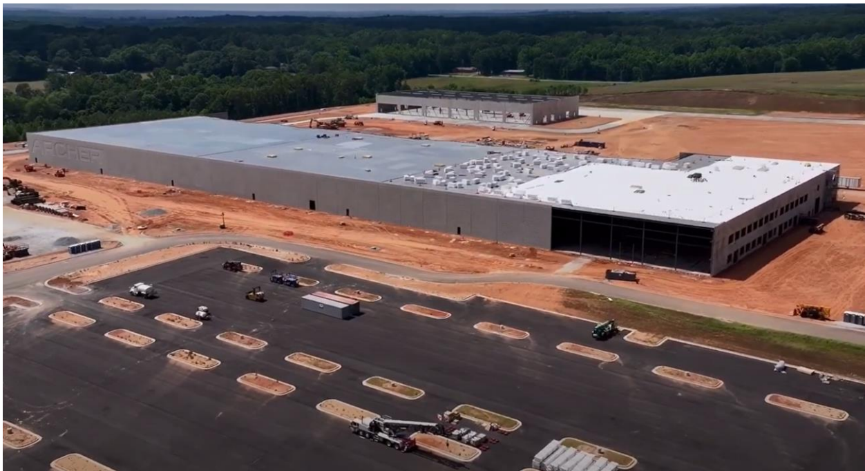
Image above shows latest progress on the construction of Archer's high-volume manufacturing facility in Covington, GA which connects to the Covington Airport
