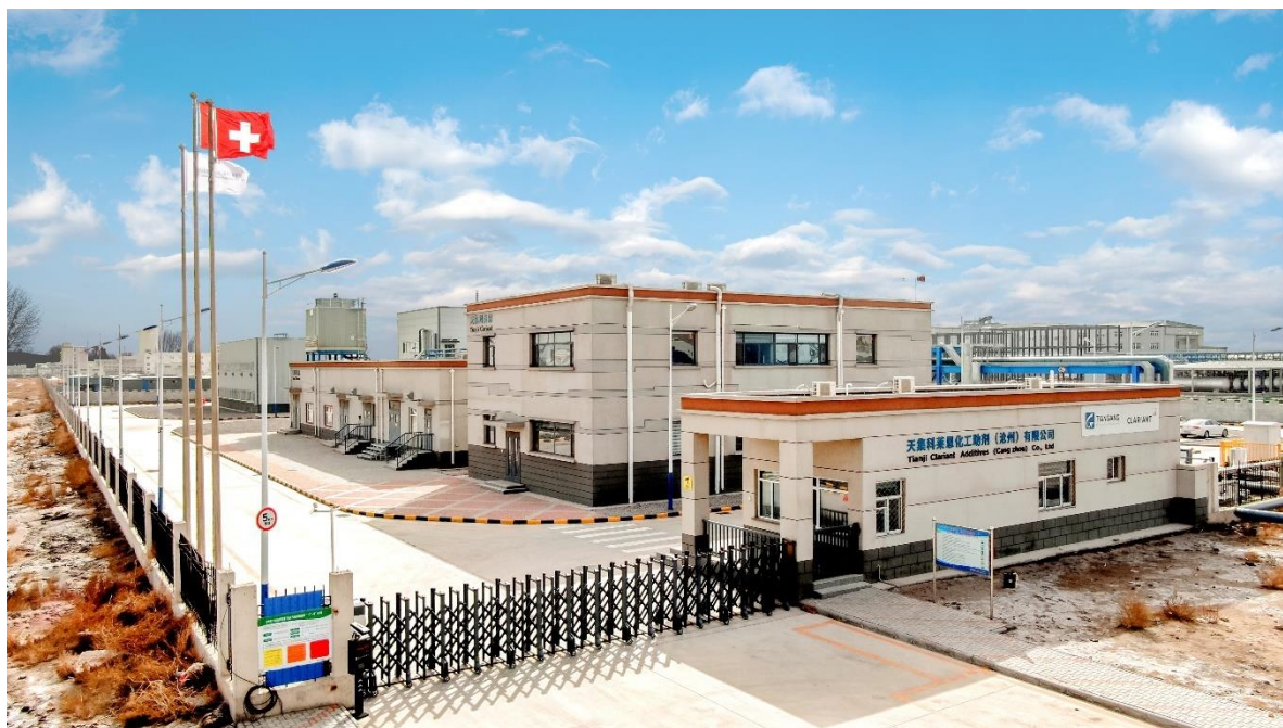
Clariant and Tiangang’s joint world-class production facility for process and light stabilizers in Cangzhou, Hebei Province (Photo: Clariant).
