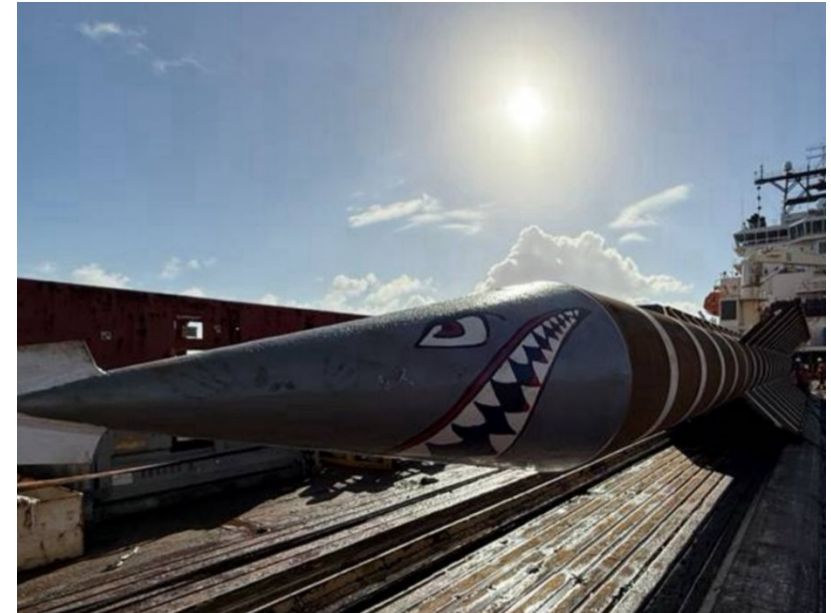
Búzios 8 torpedo installation
