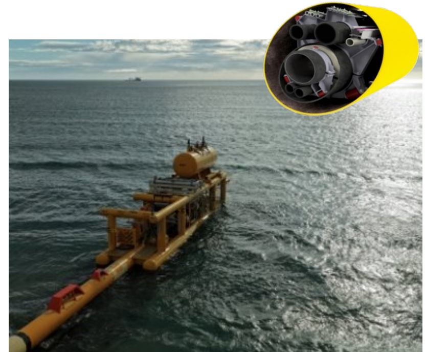
Bundle pipeline and towhead underway
