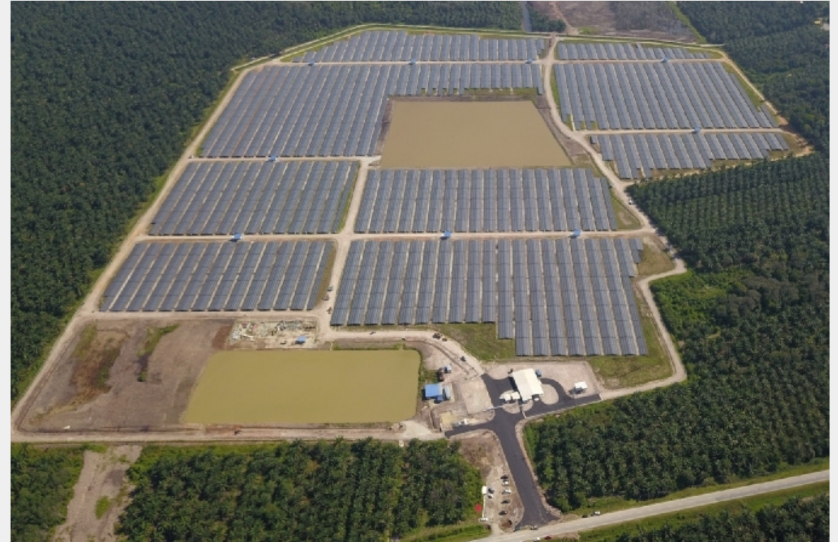
The 47 MW Redsol project in Malaysia just started commercial operations.
