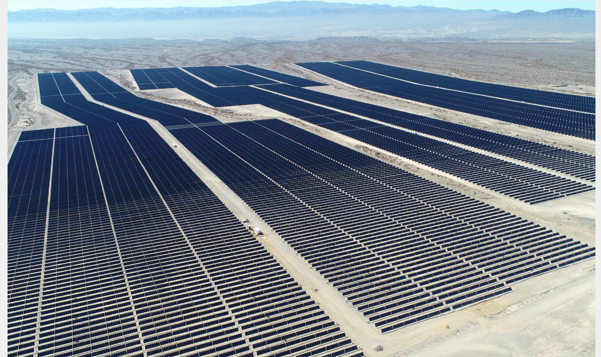
The 117 MW Guanizuil project in Argentina.
