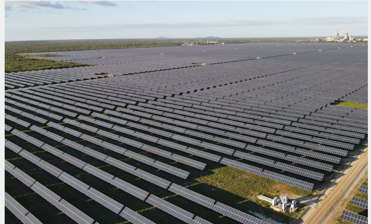
The 162 MW Apodi solar plant in Brazil.
