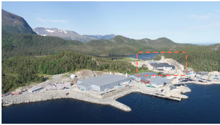
Norway - Nordheim commissioning
