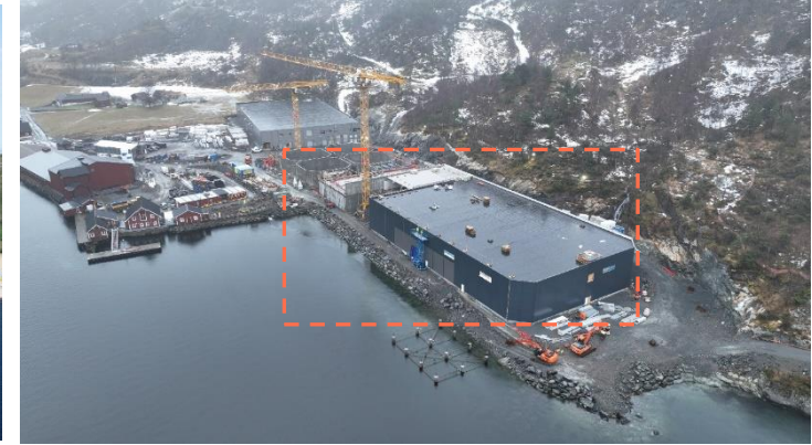
Norway - Haukå commissioning Q4-24
