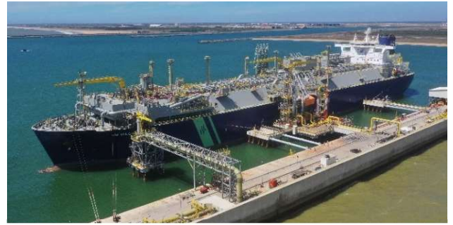
FSRU AT THE PORT OF AÇU. COURTESY BY GNA
