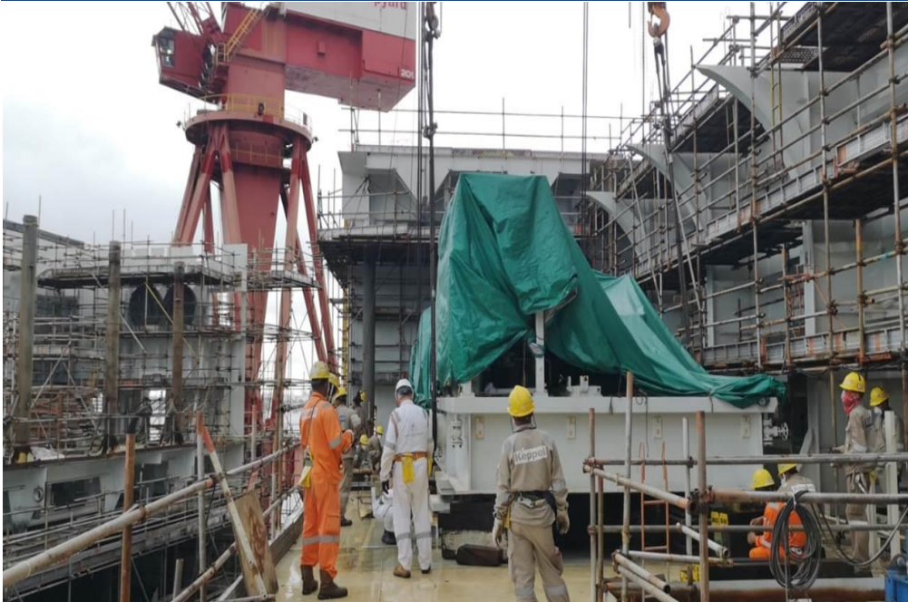
STG alternator being lifted into position within Gimi sponsons
