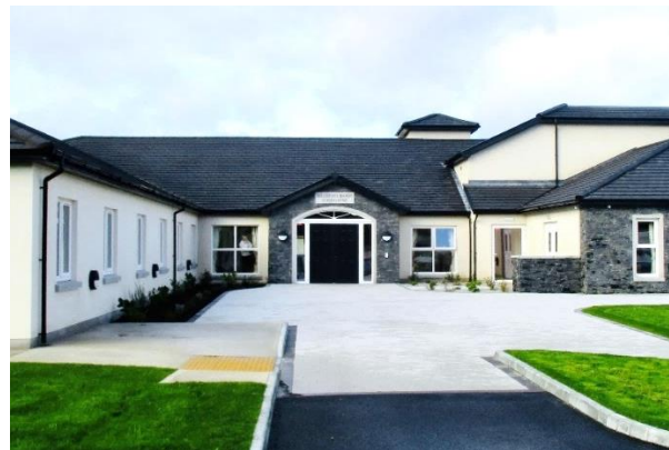
Millbrook Manor in Saggart (IE) Extension project completed in March 2023
