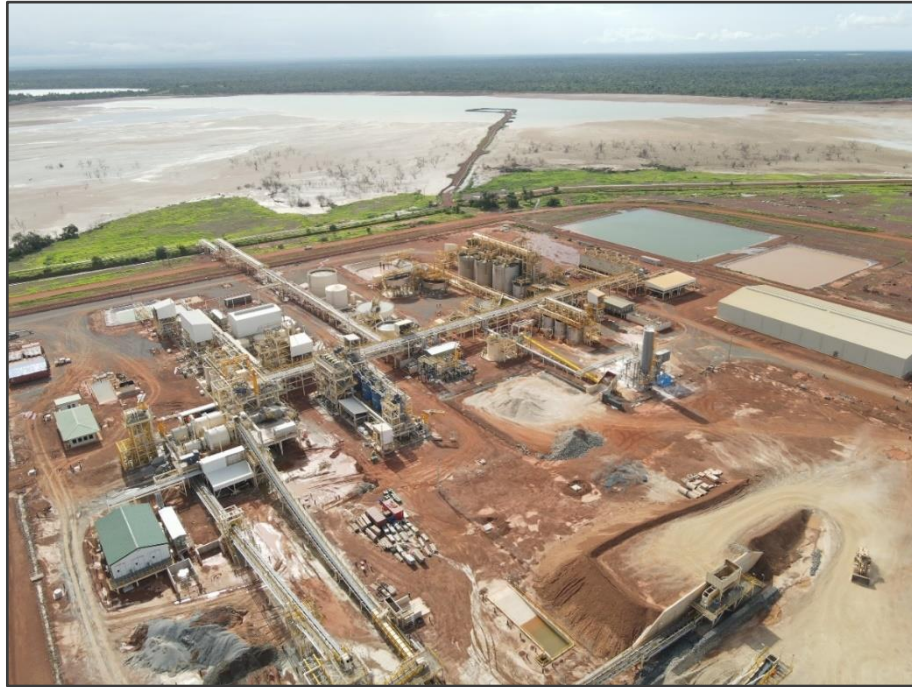
Figure 1: BIOX® processing plant overview
